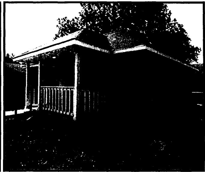
Home Reconstruction Project Taylor, Texas
