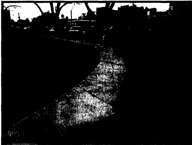
Main Street Sidewalk Improvement Project La Grange, Texas
