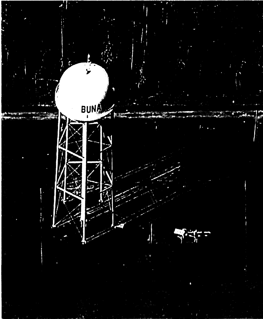
JASPER COUNTY WC & ID #1 WELL AND ELEV. TANK
